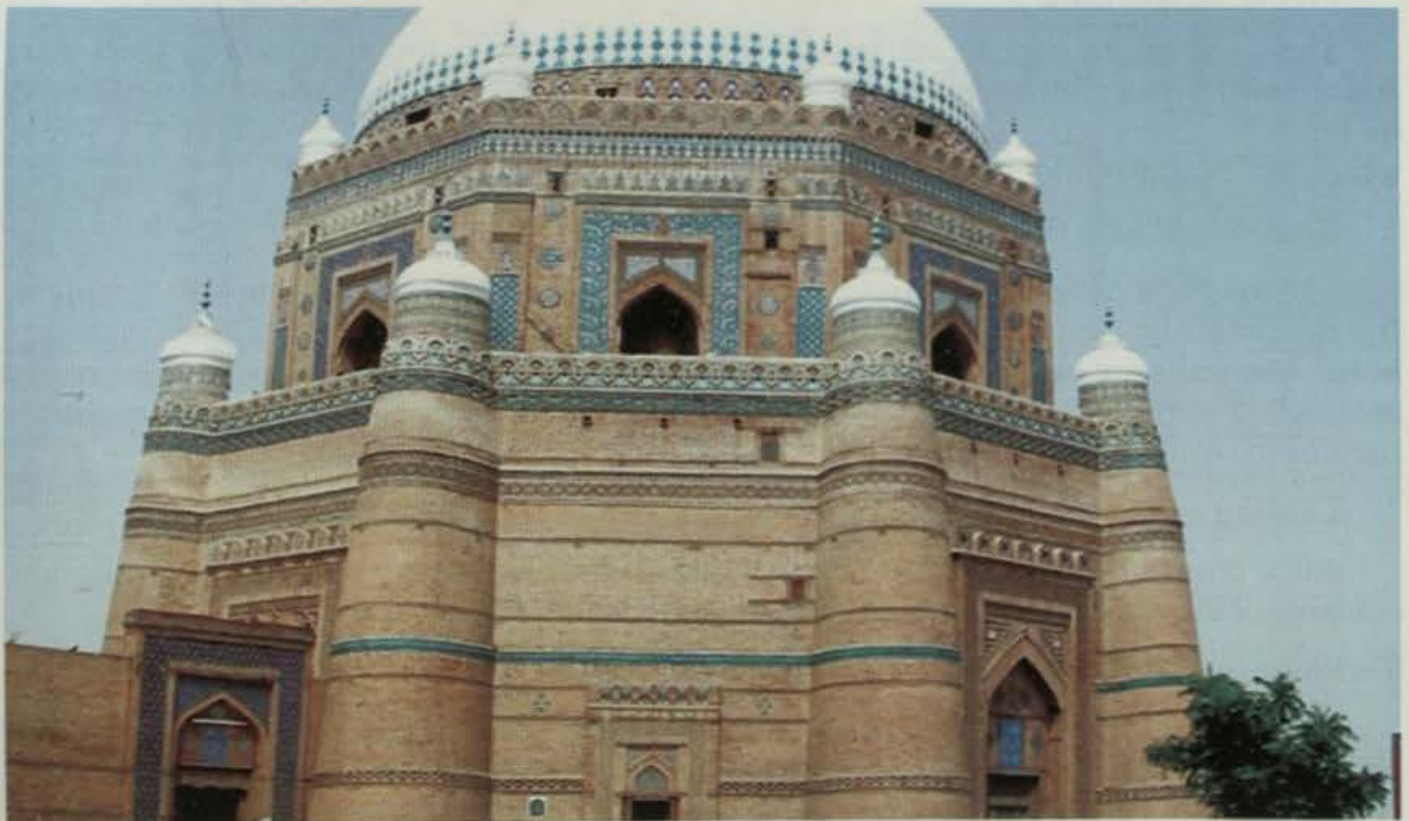
Pl. 29 Tomb of Hazrat Shah Rukn-e-Alam - Showing cut and dressed brickwork.
