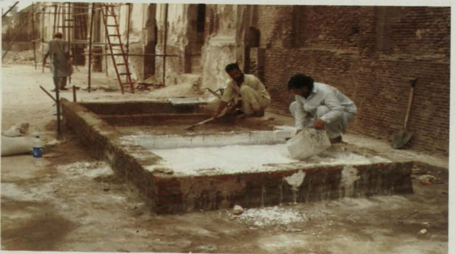
Pl. 127 Tank for slaking lime.
