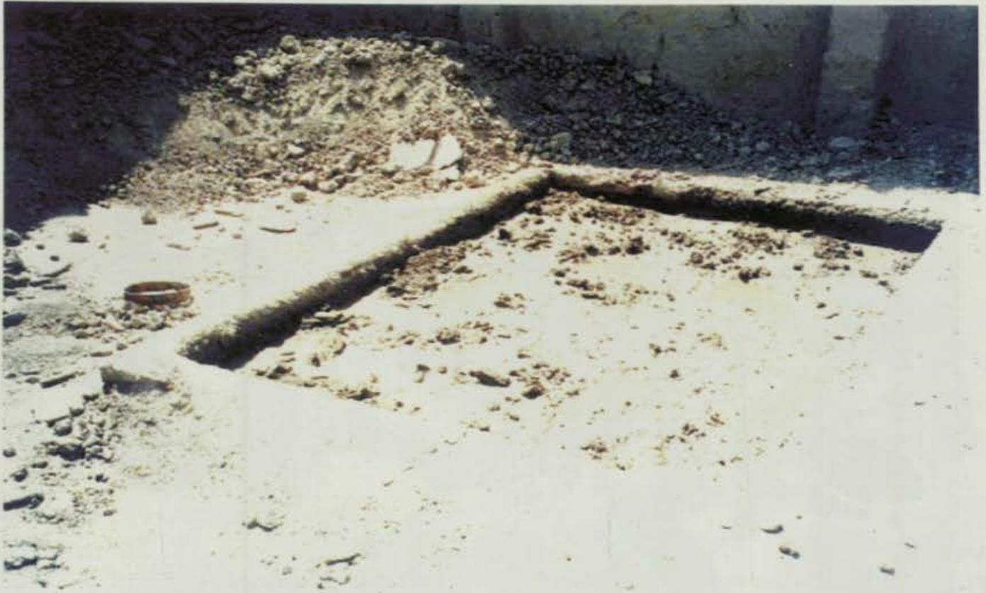
Plate. 61 Slaking of clay.
