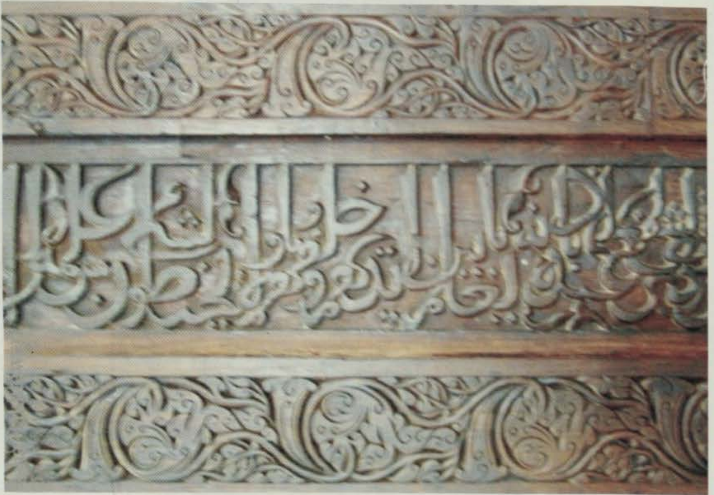
Pl. 169 Mausoleum of Hazrat Shah Rukn-e-Alam at Multan - Calligraphy work in wood.
