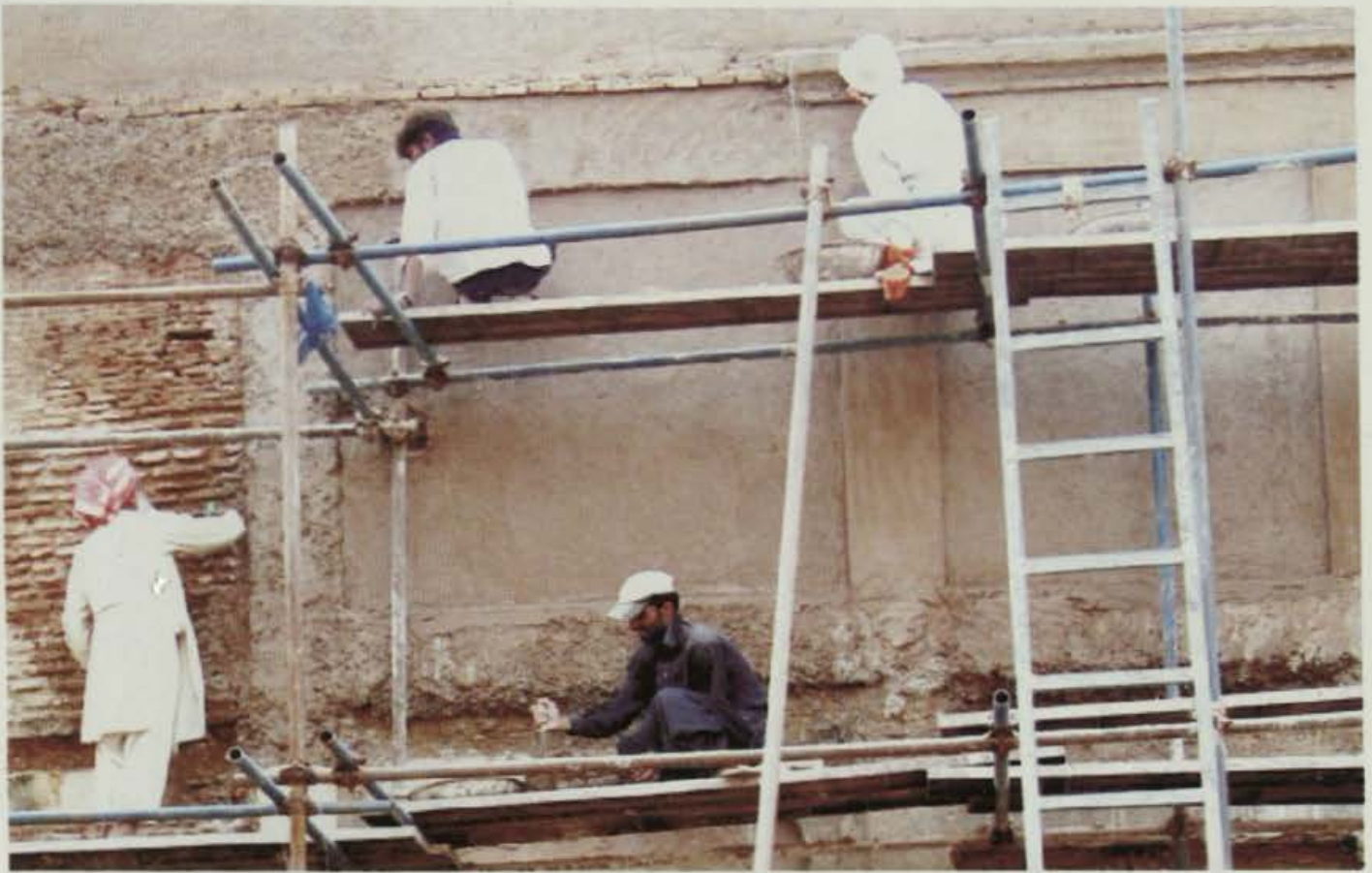
Pl. 131 Applying kankar lime plaster.
