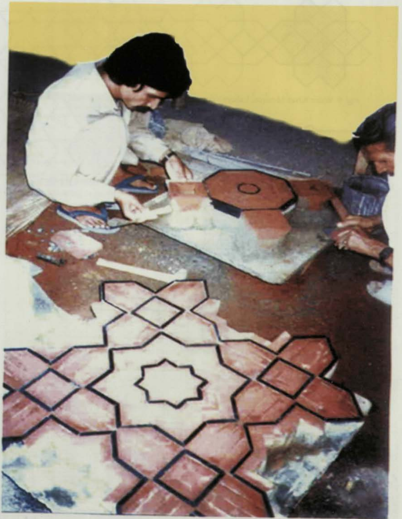
Pl. 41 Laying of cut and dressed brick flooring in geometrical pattern.
