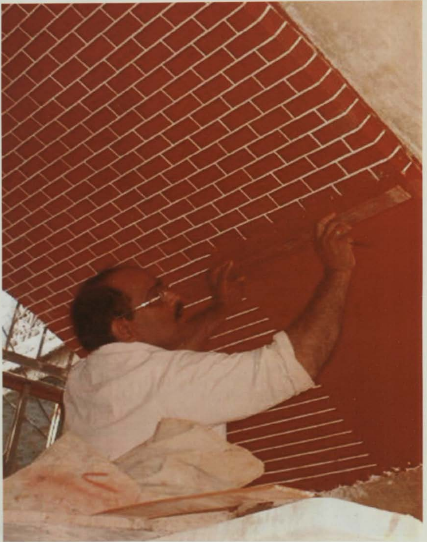
Pl. 142 Brick Imitation work in progress on soffit of arch.
