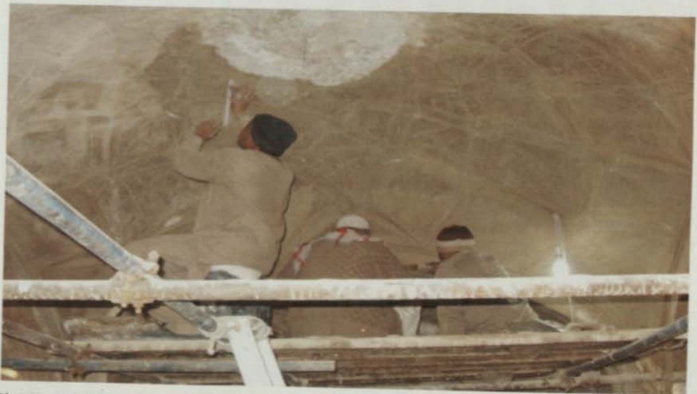
Pl. 168 Ghalib kari (stalactite work) in progress.
