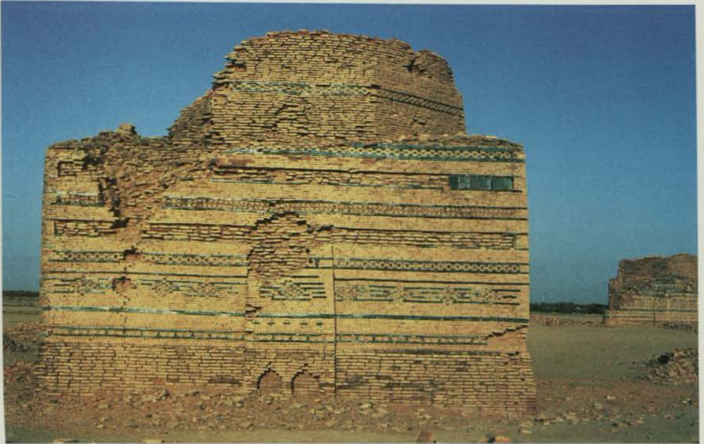
Pl. 28 Temple Sassi- da -Kallara at Shah Muhammad Wali, Attock - Showing cut and dressed brickwork.
