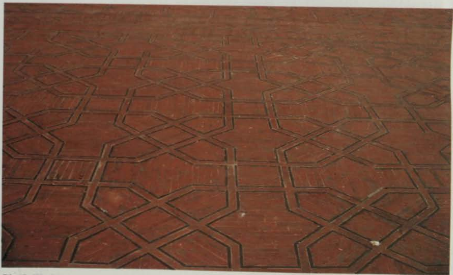
Pl. 40 Wazir Khan Mosque, Lahore - Showing cut and dressed brick floor.
