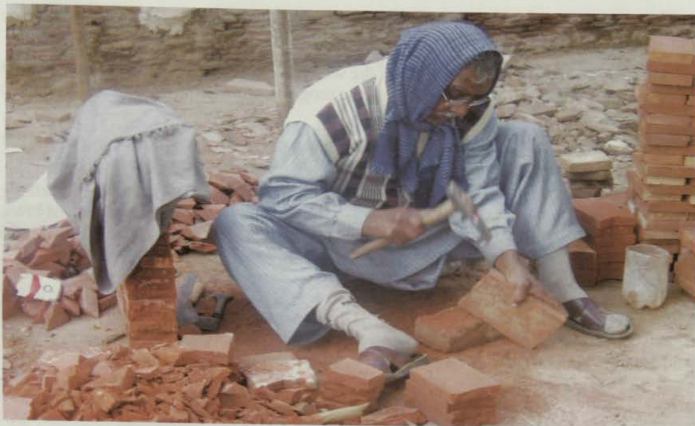
Pl. 33 Dressing and cutting of brick.s.
