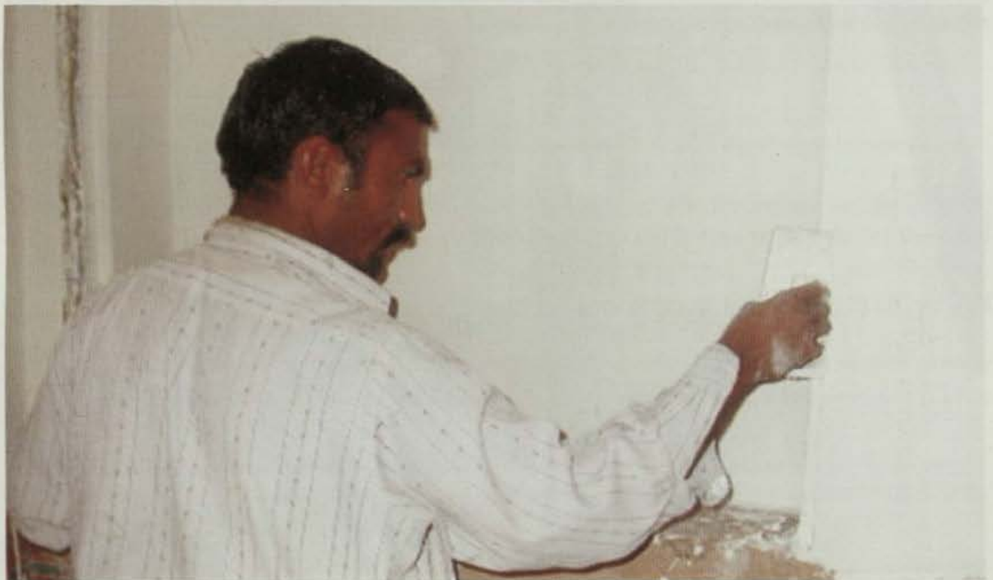
Pl. 132 Applying glazed lime plaster.
