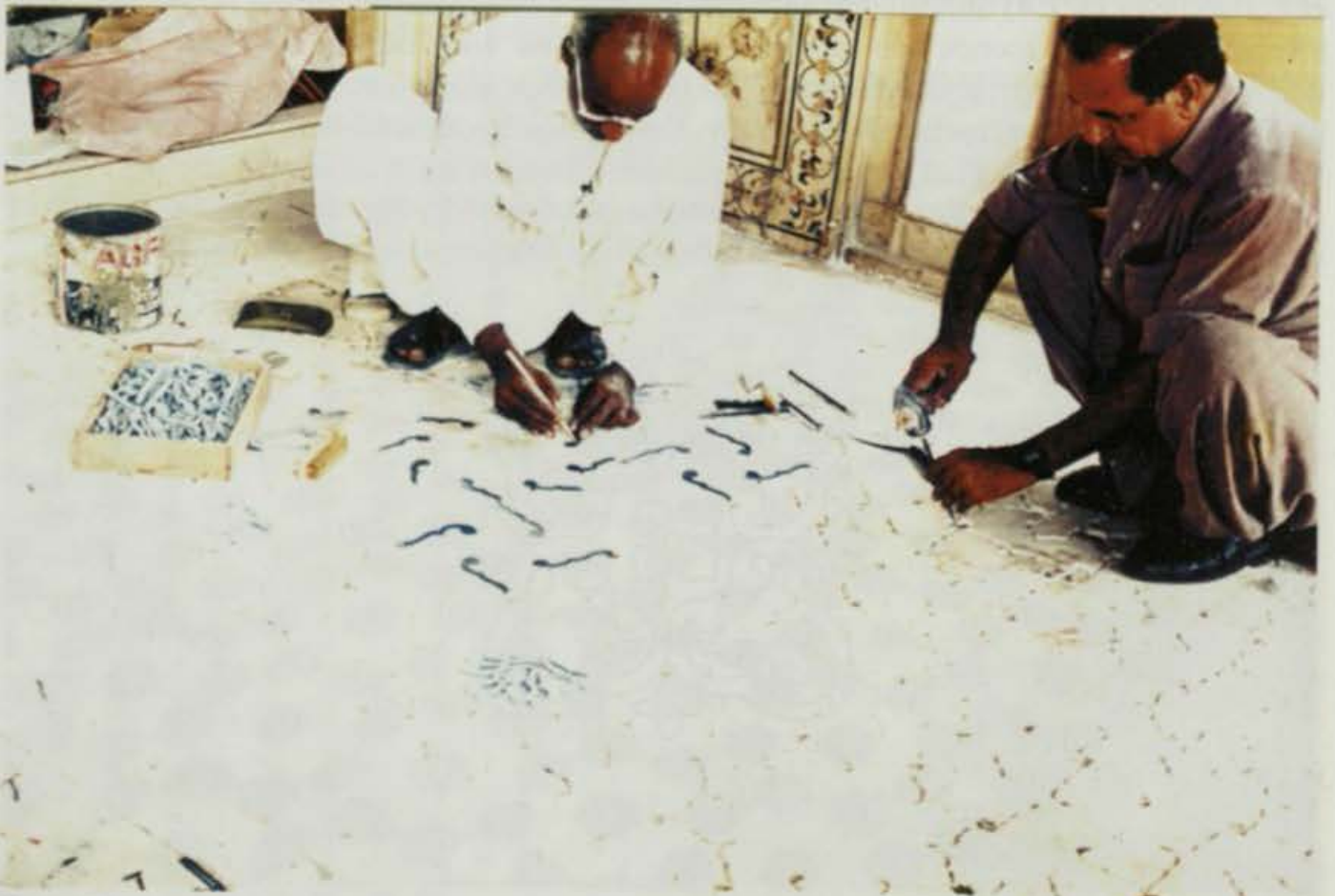
Pl. 106 Laying of tessellated floor.
