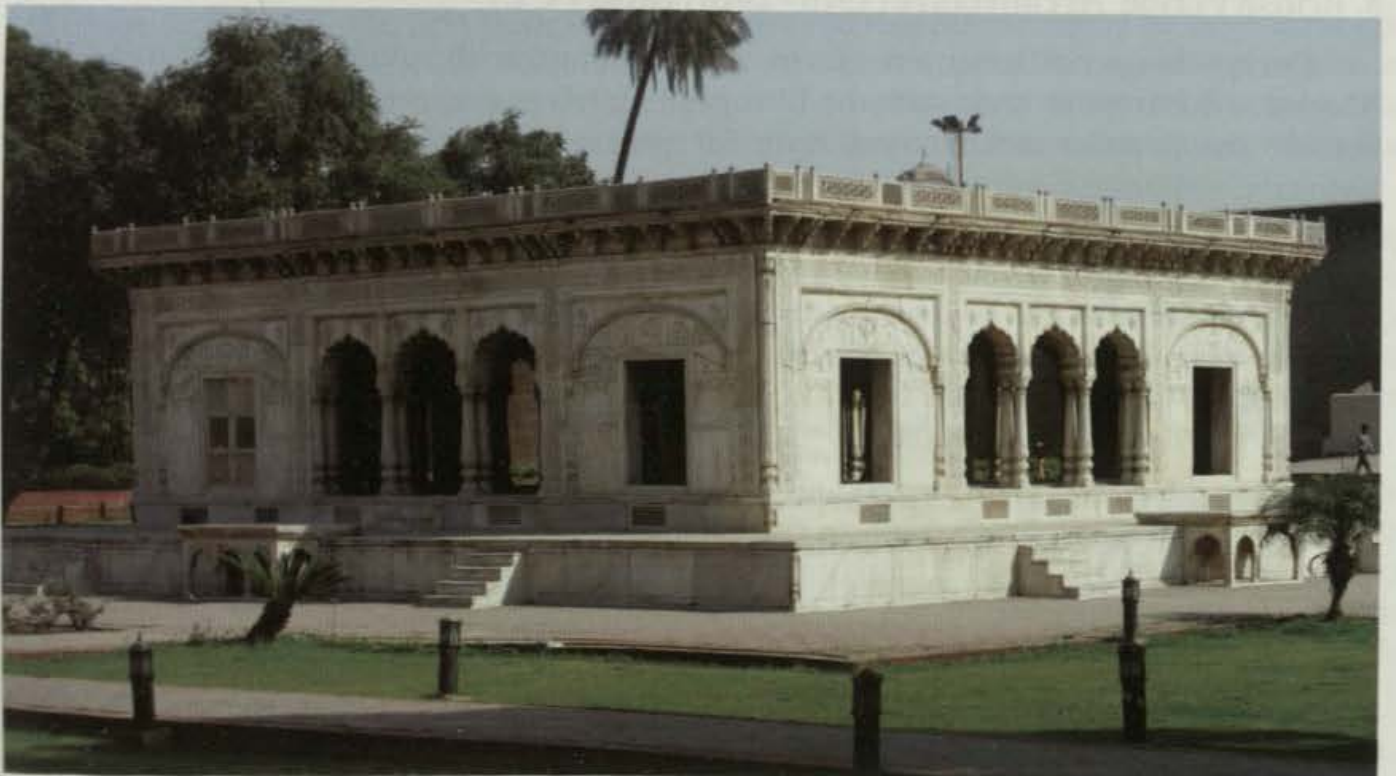
Pl. 24 Baradari in Hazoori Bagh, Lahore - General view.
