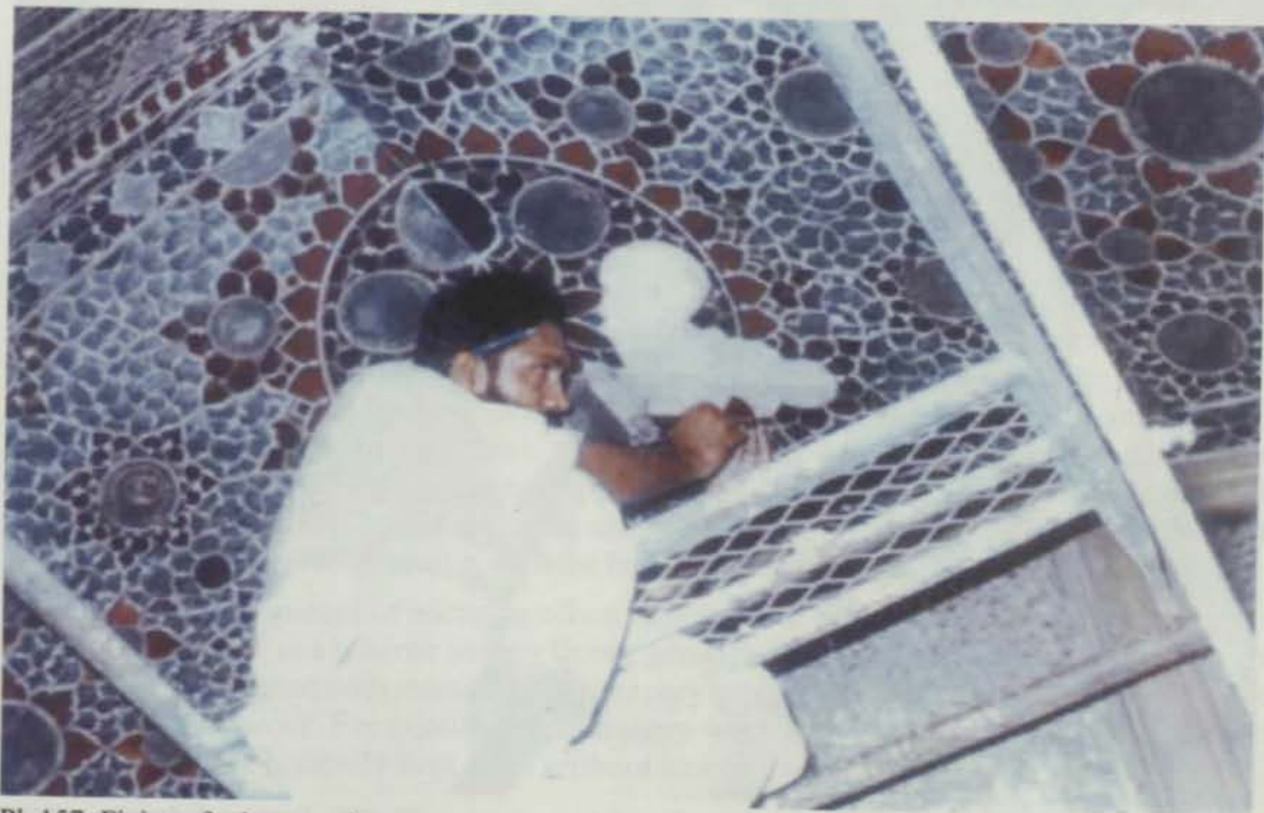
Pl. 157 Fixing of mirror work.
