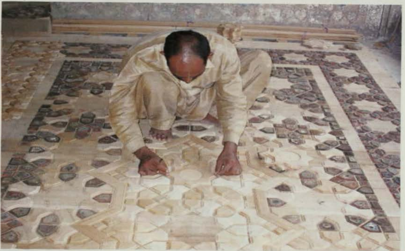
Pl.123 Preparing of wooden panel in Tarseen Bandi .
